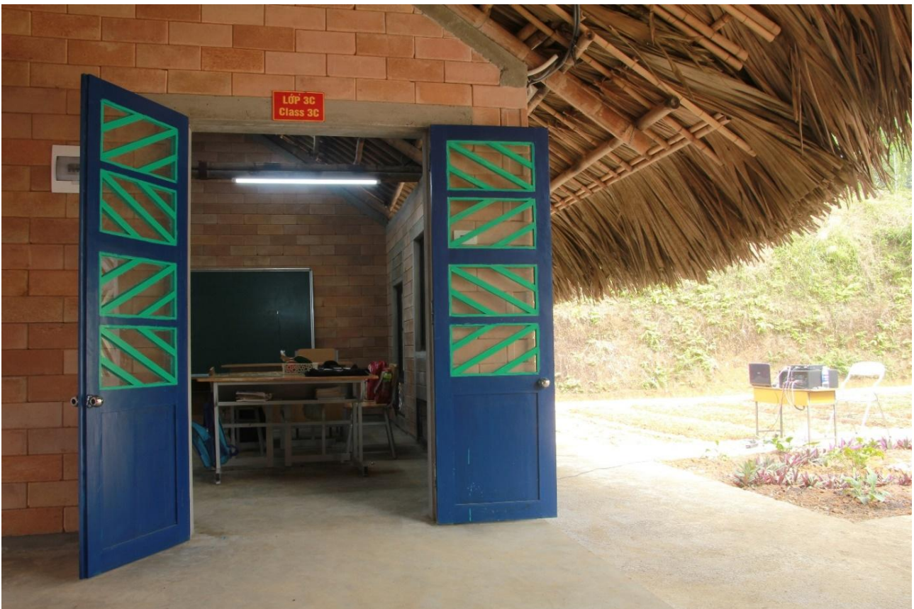
Overhang thatched roof provide high sun shading and keep room longer cooler in summer
