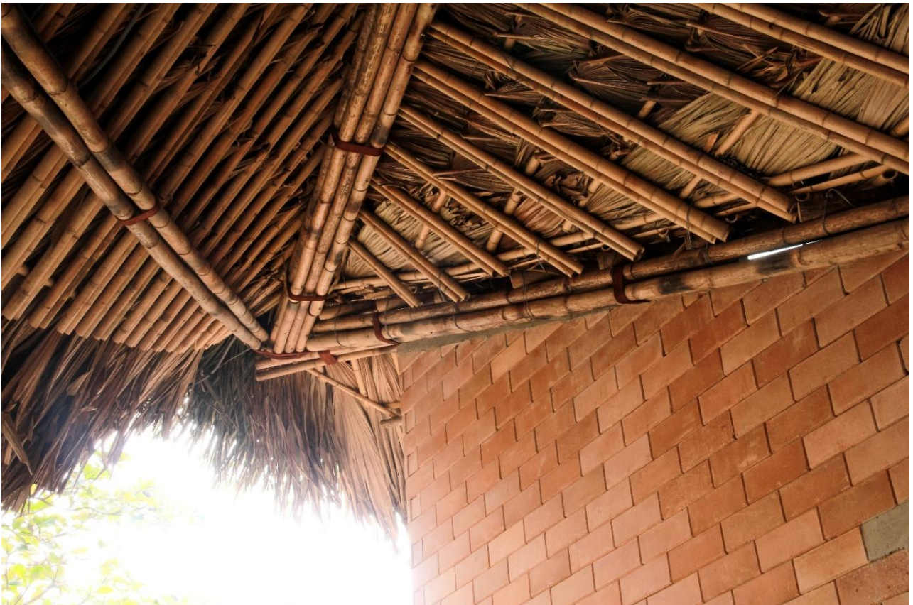
Bamboo frame with over 4000 dried leaves collected from near mountains
