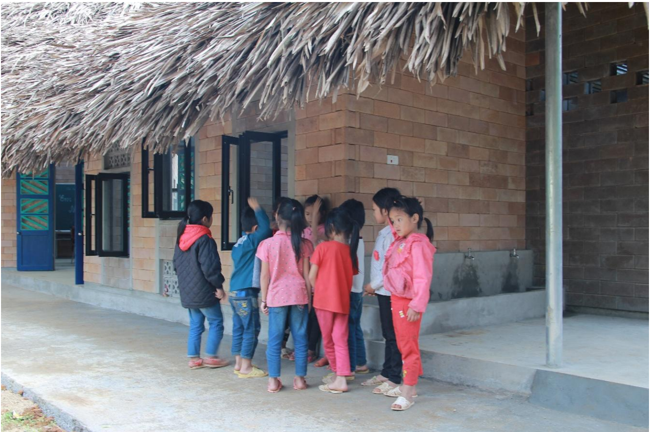
Windows with ventilation bricks
