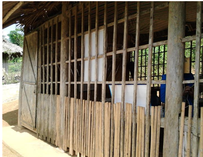
The classroom envelope is only a wooden frame structure which not function for a thermal comfort in summer and winter.
