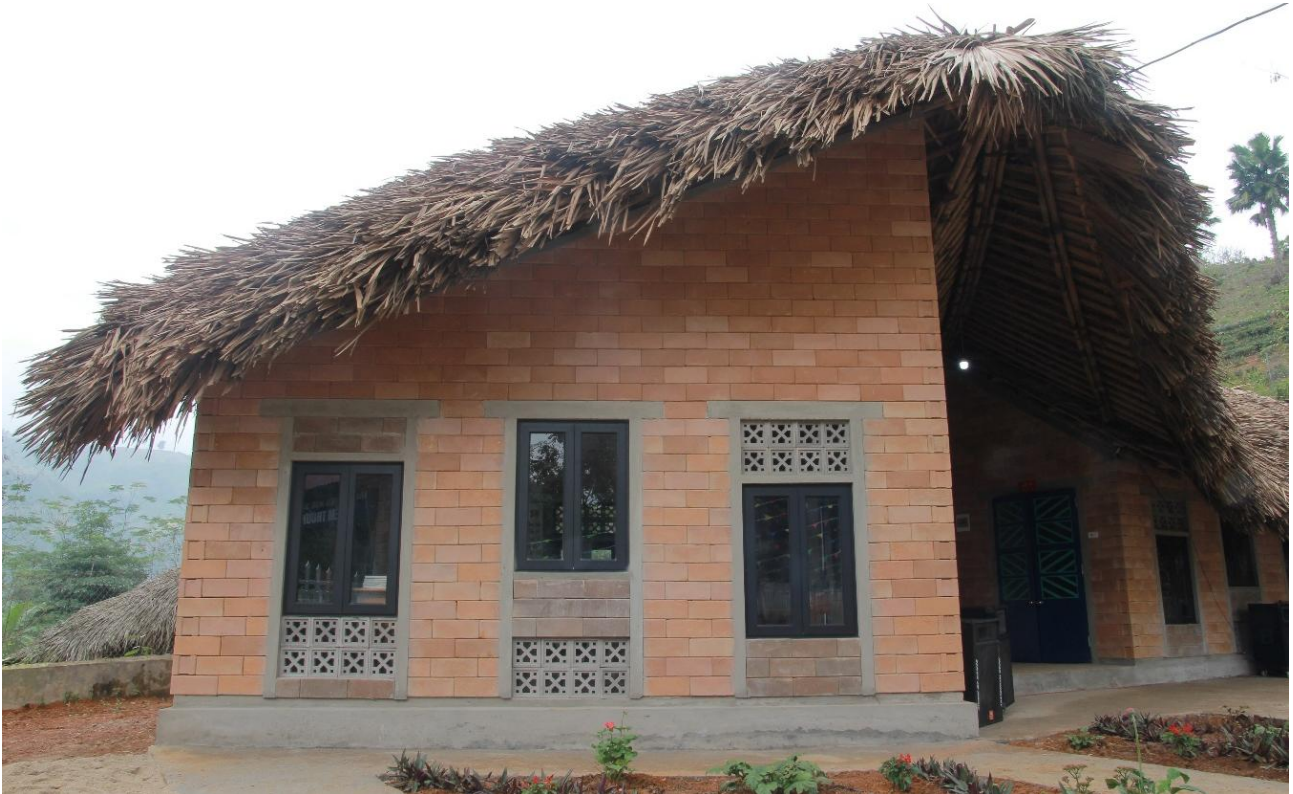
Windows with ventilation bricks
