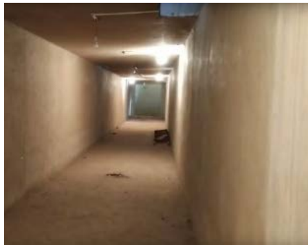
Image 1: Underground earth duct
