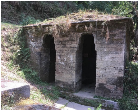
Photo 4: Water is found a Naula, as shown here in this photo. A naula is a traditional water harvesting system, usually found at the roots of a scared oak tree. Here you can see a small temple constructed over it.
