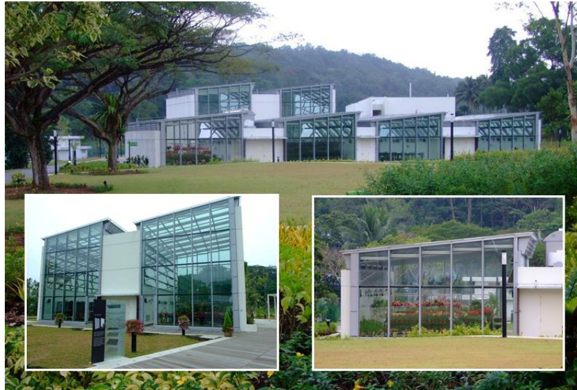
Figure 2: 6 Prototypes to test façade, envelope and mechanical strategies. 2 high prototypes to test stratification and removal of solar gains by cross ventilation. 4 prototypes with different high selective glazing and ventilation systems. Client: National Parks Singapore. Design Team: Architect: Nirmal Kishnani and CPG; MEP: CPG; Structure: CPG.
