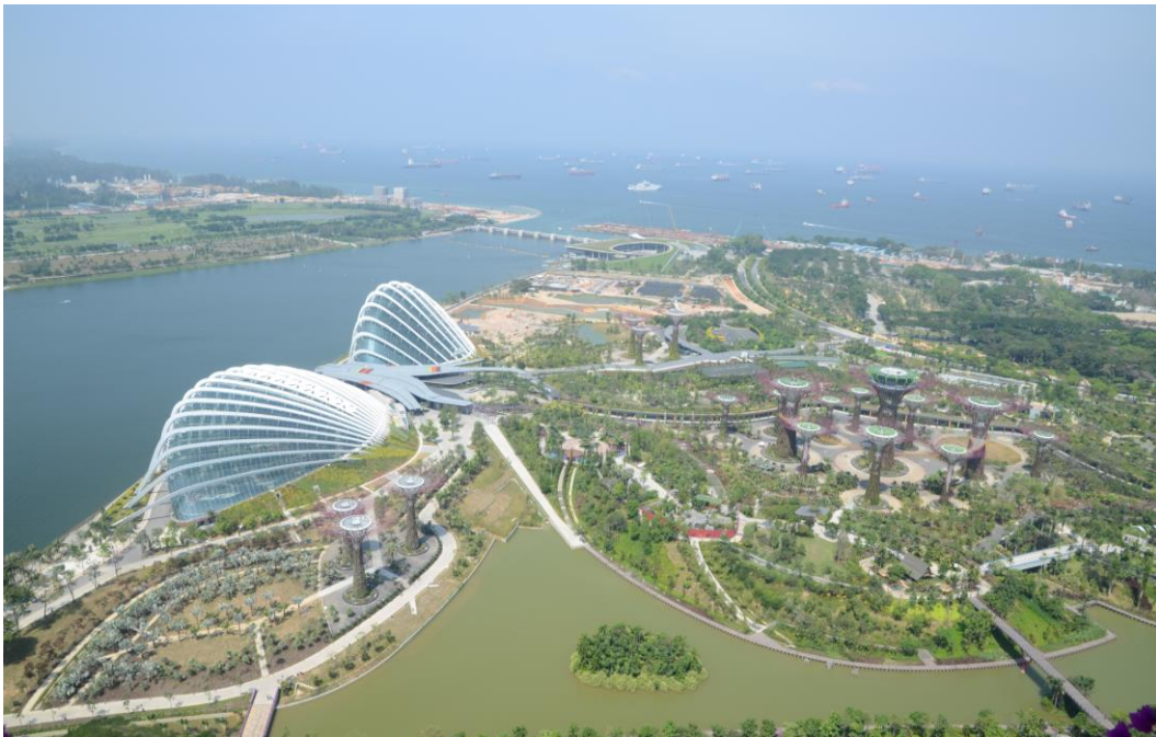
Figure 1: Cooled Conservatories at the Gardens by the Bay, Singapore designed by Wilkinson Eyre, London Client: National Parks Singapore. Design Team: Architect: Wilkinson Eyre and CPG; VAC: atelier ten and CPG; Structure: atelier one and CPG; Landscape: Grant Associates.
